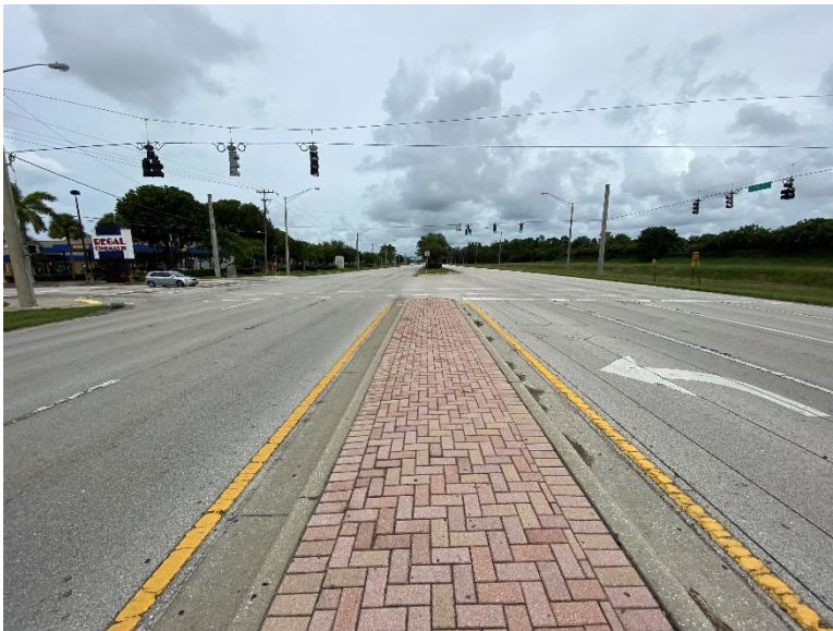
SR-7 looking north near the signalized intersection at Regal Cinemas 18.
