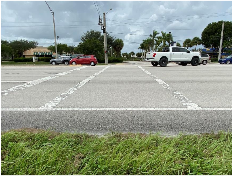
Crosswalk on the south side of the Regal 18 Cinemas signalized intersection does not lead to a sidewalk on the east side, looking west.
