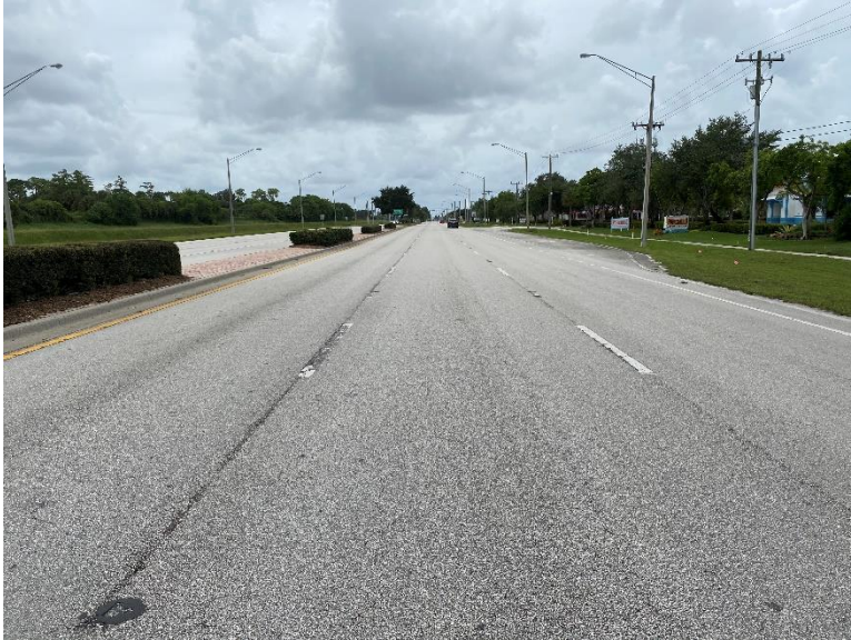
SR-7 between Belvedere Rd and Okeechobee Blvd has three (3) through lanes in each direction as shown here in the southbound lanes looking south.
