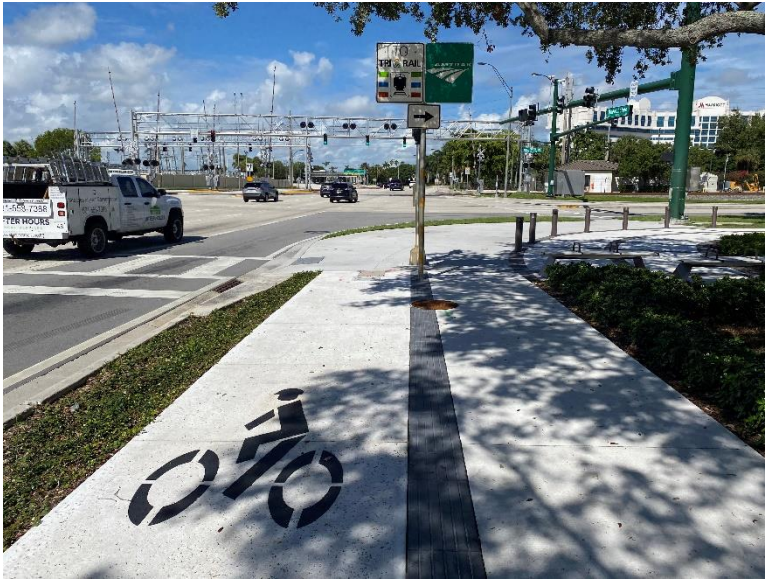
Westbound raised separated bicycle lane adjacent to sidewalk on the north side of Okeechobee Blvd east of Tamarind Avenue looking west.
