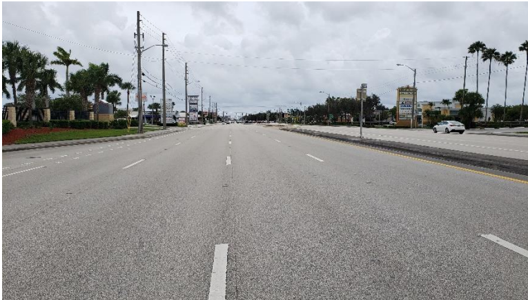
Westbound four (4) through lanes of Okeechobee Blvd looking east near Military Trail.
