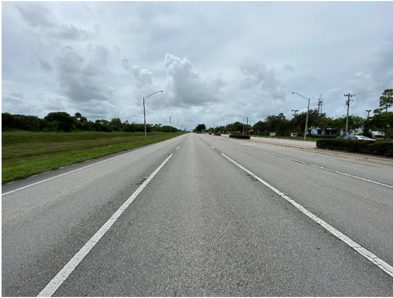
Northbound through lanes and a left-turn lane south of the Regal Cinemas 18 intersection looking south.
