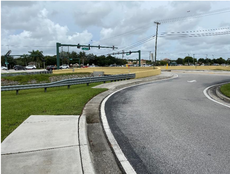
Short section of missing sidewalk in the Buckingham Square shopping center driveway on the east side of SR-7 south of Pioneer Road.
