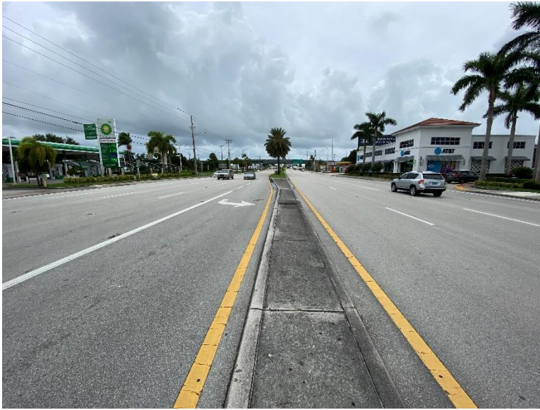
Traffic separator median on Okeechobee Blvd looking east at the westbound left-turn lane to the Palm Beach Marketplace shopping center.
