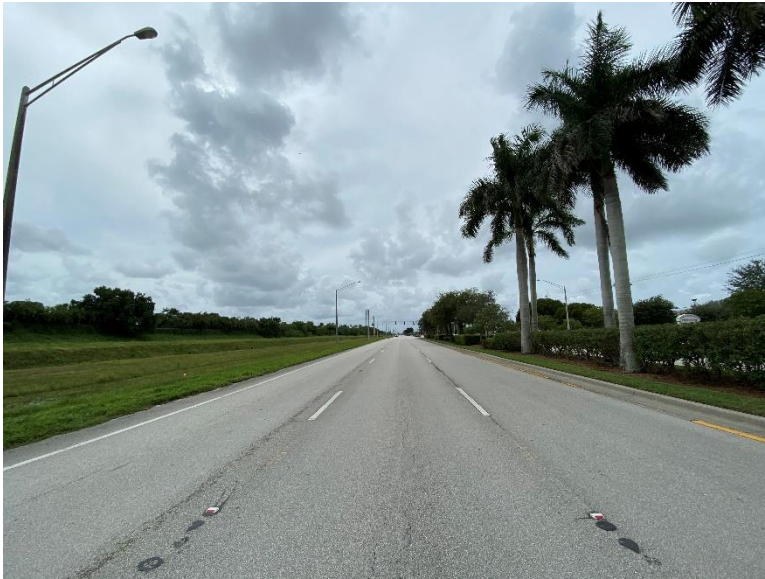
Northbound three (3) through lanes looking south.
