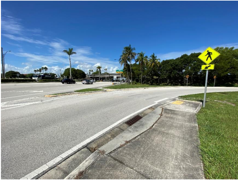
The crosswalk on the north side of Okeechobee Blvd across the Australian Avenue northbound on-ramp looking west.
