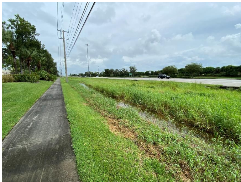
West side of SR-7 looking north with existing 5 feet wide sidewalk and drainage swale separating pedestrians and motorists.
