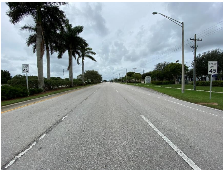
Southbound three (3) through lanes looking south.
