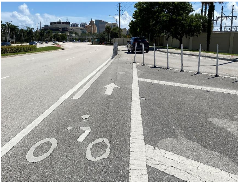
The eastbound bicycle lane approaching the ramp from Australian Avenue to eastbound Okeechobee Blvd includes flexible traffic delineator posts.
