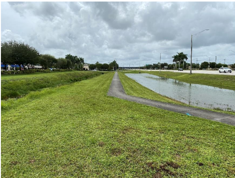
The sidewalk on the east side of SR-7 south of Weisman Way looking south, which exists between a canal to the left and a drainage swale to the right.
