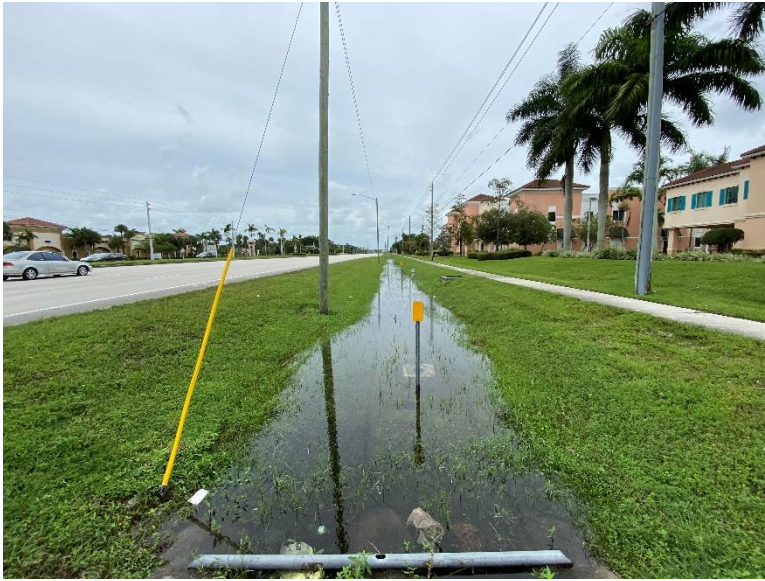
The north side sidewalk is separated from the roadway by a drainage swale looking west.
