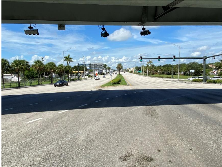
Okeechobee Blvd looking west under the I-95 southbound flyover ramp.
