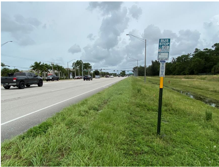
Bus stops exist on the east side of SR-7 in this section but with no sidewalks, such as at Bus Stop # 3472.
