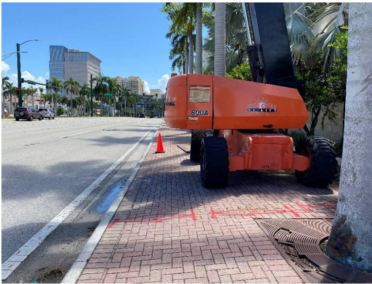
A maintenance crane blocking the sidewalk outside of the Convention Center on the south side of Okeechobee Blvd.
