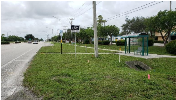
A typical Palm Tran bus stop along SR-7 in this area includes seating area with shelter and a 5 feet wide sidewalk connecting to the road. A pipe culvert exists to carry the drainage swale under the sidewalk.
