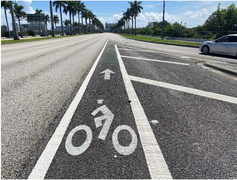
The eastbound bicycle lane is not buffered and includes a crossing of high-speed traffic from northbound I-95 to eastbound Okeechobee Blvd.
