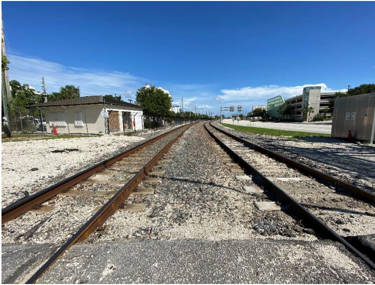
The South Florida Rail Corridor (SFRC) crossing looking north.
