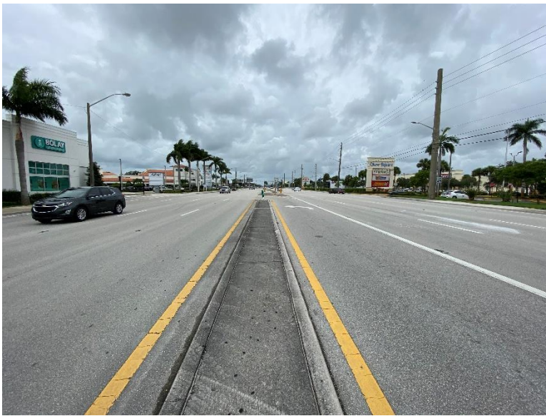
Traffic separator median on Okeechobee Blvd looking west at the westbound left-turn lane to the Palm Beach Marketplace shopping center.
