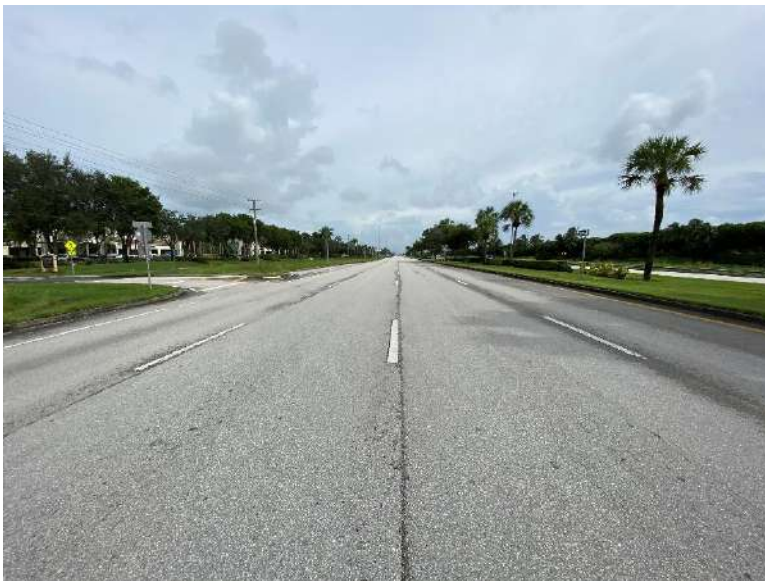
Four (4) southbound through lanes along SR-7 looking north.
