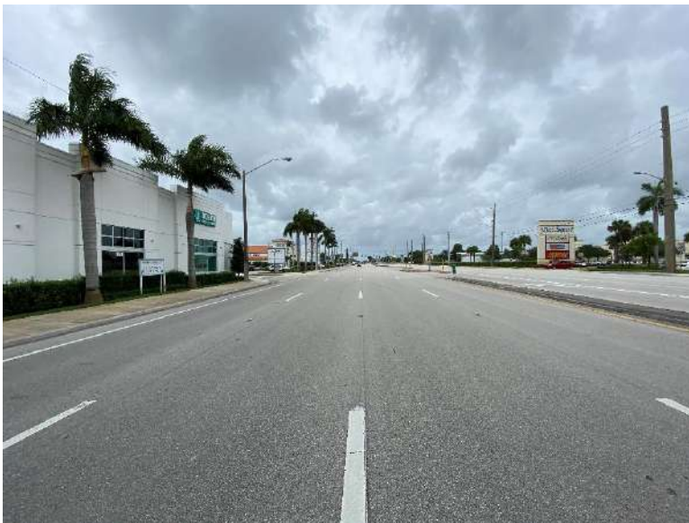
Eastbound four (4) through lanes of Okeechobee Blvd looking west near Church Street.
