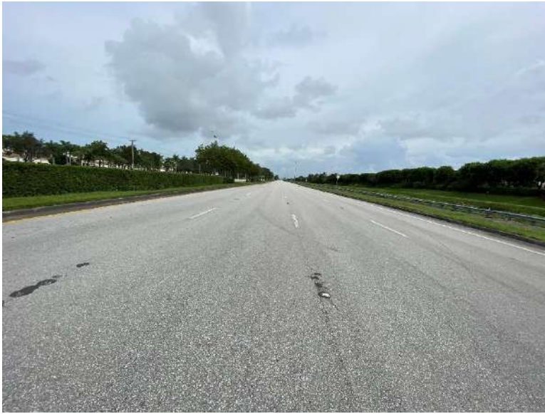
Four (4) northbound through lanes along SR-7 looking north.
