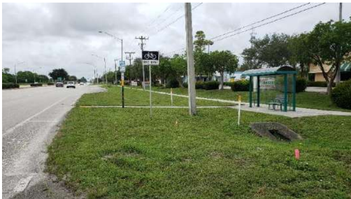
A typical Palm Tran bus stop along SR-7 in this area includes seating area with shelter and a 5 feet wide sidewalk connecting to the road. A pipe culvert exists to carry the drainage swale under the sidewalk.
