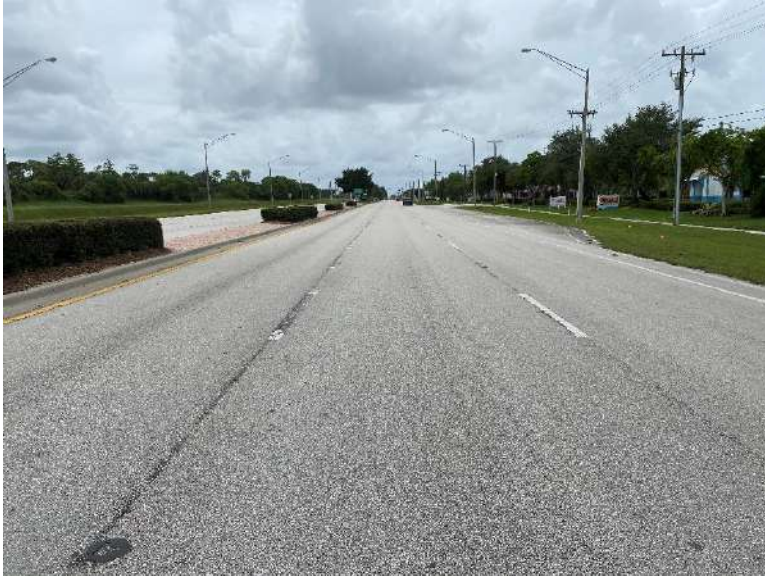
SR-7 between Belvedere Rd and Okeechobee Blvd has three (3) through lanes in each direction as shown here in the southbound lanes looking south.
