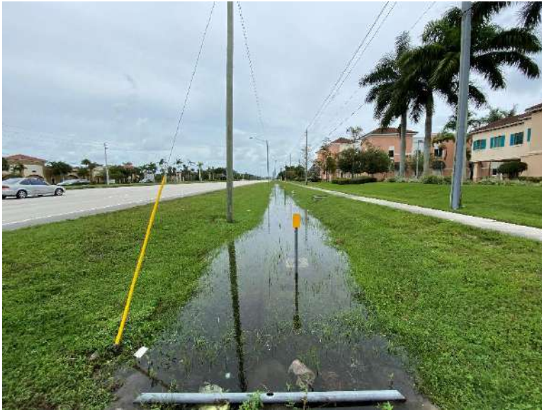
The north side sidewalk is separated from the roadway by a drainage swale looking west.
