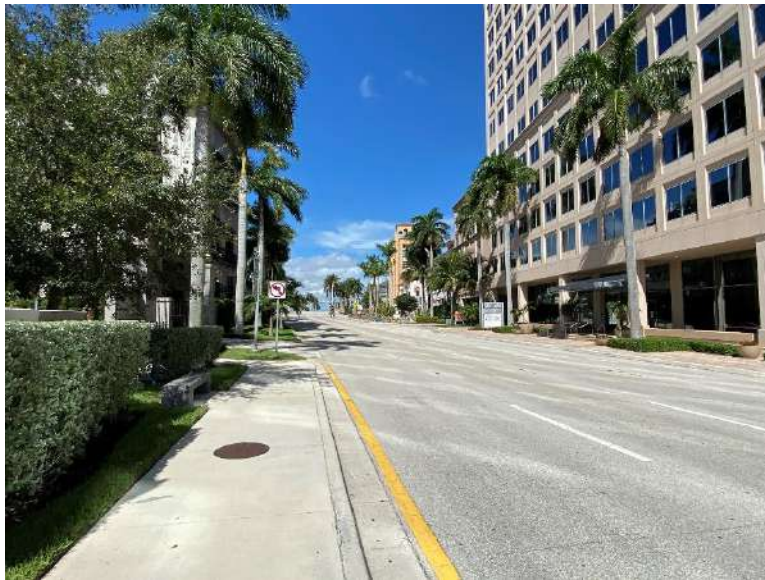
SR-704 is a one-way pair between Rosemary Avenue and US-1, with four (4) westbound lanes carried by Lakeview Avenue looking west.
