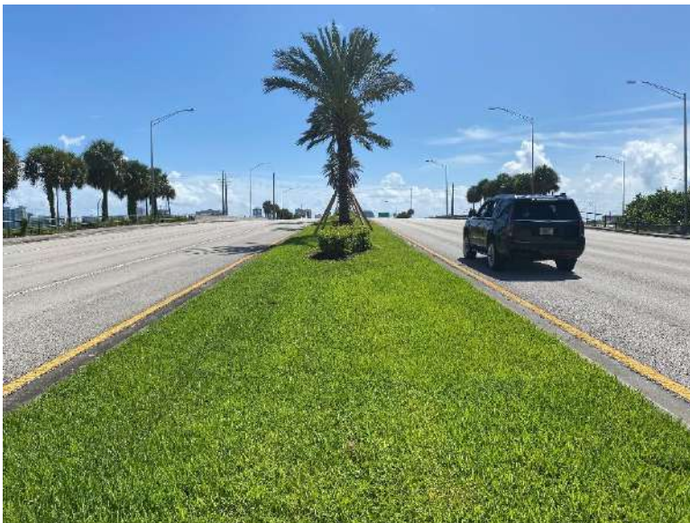
Okeechobee Blvd median looking east on the approach to the I-95 overpass.
