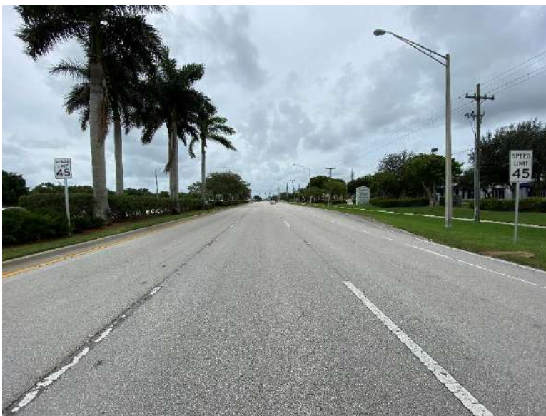
Southbound three (3) through lanes looking south.
