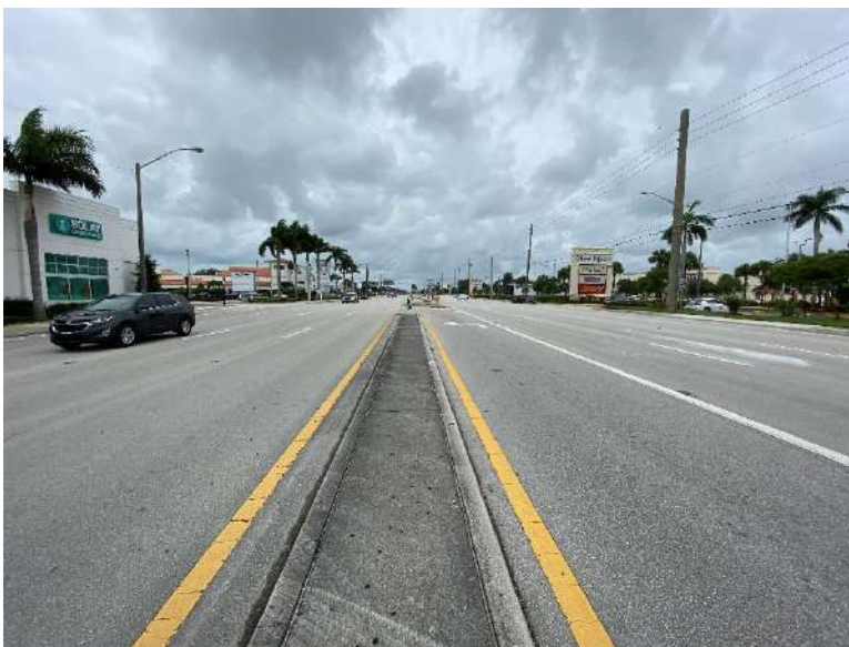
Traffic separator median on Okeechobee Blvd looking west at the westbound left-turn lane to the Palm Beach Marketplace shopping center.
