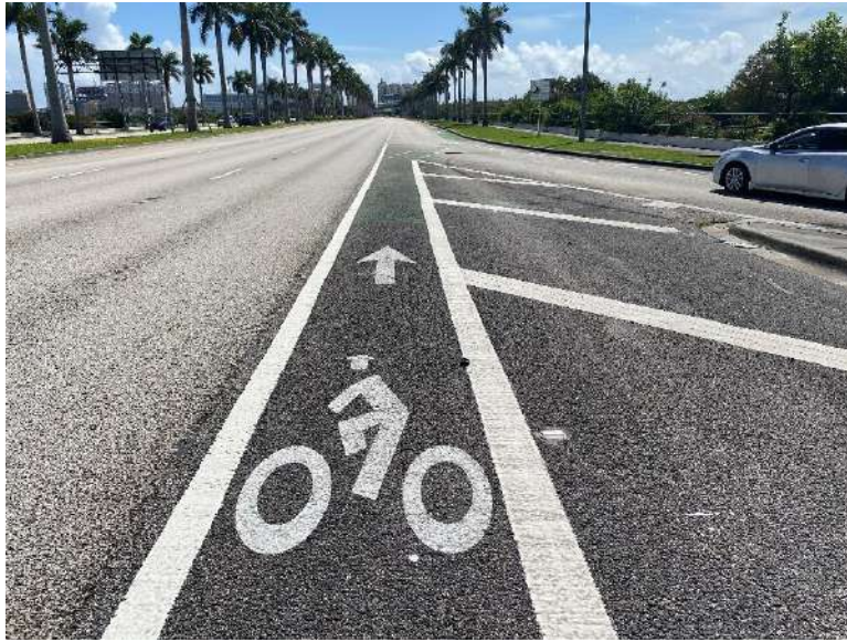
The eastbound bicycle lane is not buffered and includes a crossing of high-speed traffic from northbound I-95 to eastbound Okeechobee Blvd.
