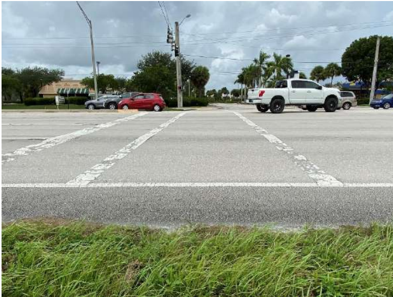
Crosswalk on the south side of the Regal 18 Cinemas signalized intersection does not lead to a sidewalk on the east side, looking west.
