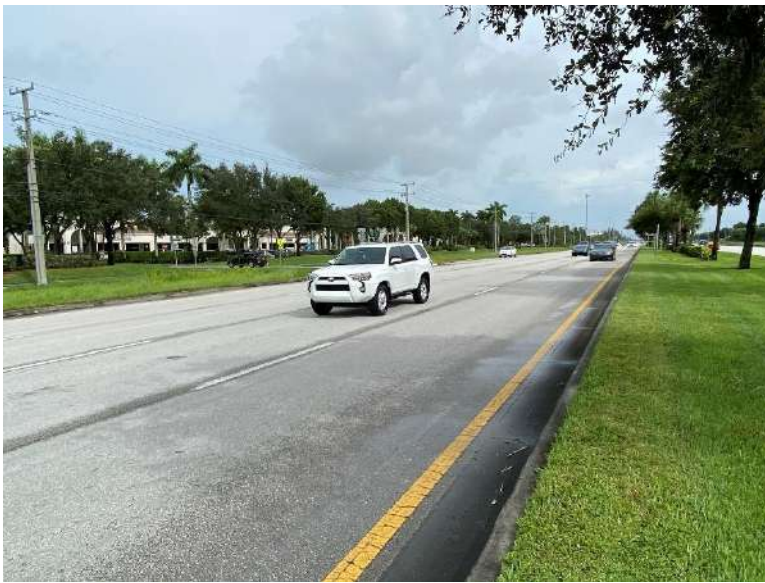
Traffic in four (4) southbound through lanes on SR-7 looking north.
