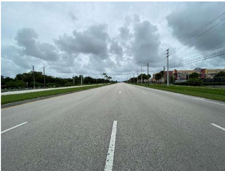
Eastbound four (4) through lanes of Okeechobee Blvd looking east near Turning Points Academy School.
