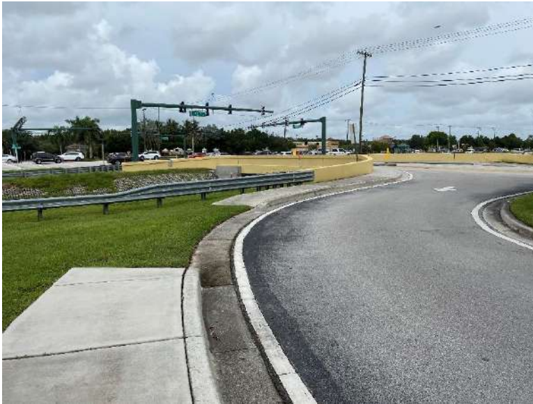
Short section of missing sidewalk in the Buckingham Square shopping center driveway on the east side of SR-7 south of Pioneer Road.
