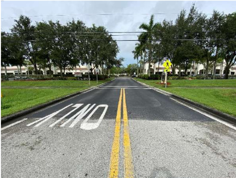
The wide offset between the west sidewalk and the roadway creates midblock crosswalks at driveways.
