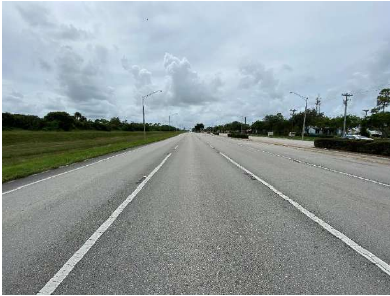
Northbound through lanes and a left-turn lane south of the Regal Cinemas 18 intersection looking south.
