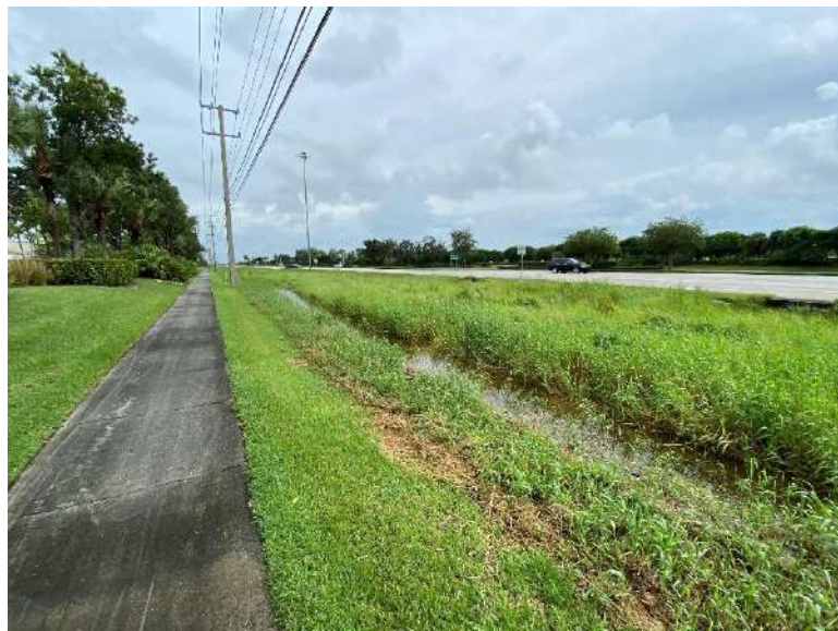
West side of SR-7 looking north with existing 5 feet wide sidewalk and drainage swale separating pedestrians and motorists.
