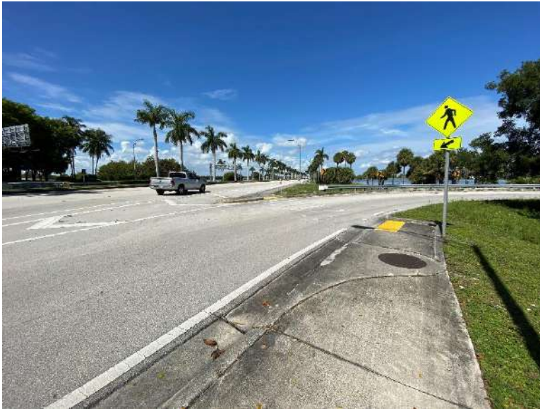
The crosswalk on the north side of Okeechobee Blvd across the Australian Avenue southbound on-ramp looking west. The Australian Avenue interchange is a partial cloverleaf, which presents challenges for pedestrians and bicyclists.
