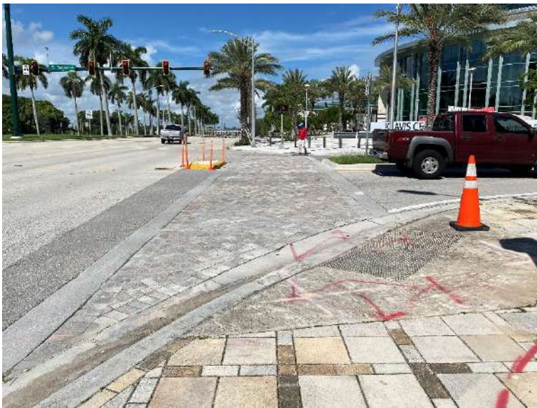
Crosswalk across Sapodilla Avenue on the north side of Okeechobee Blvd looking west.
