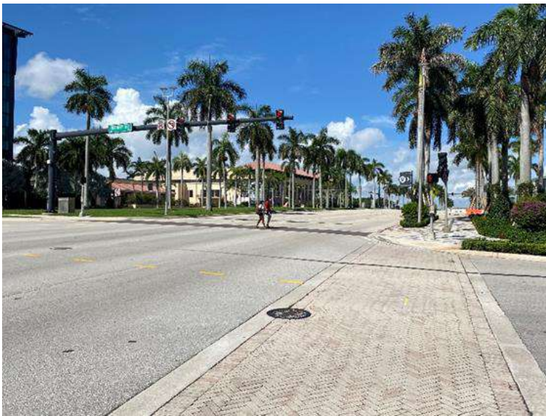
Crosswalk across Rosemary Avenue on the north side of Okeechobee Blvd looking west.
