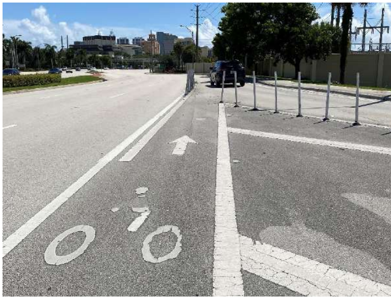
The eastbound bicycle lane approaching the ramp from Australian Avenue to eastbound Okeechobee Blvd includes flexible traffic delineator posts.
